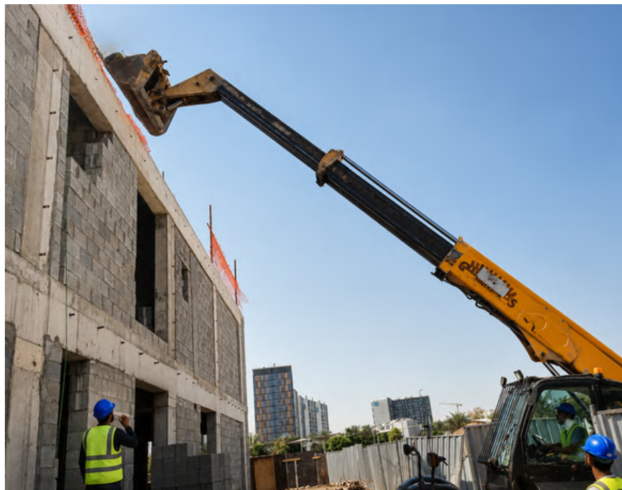
Construction of Villa in Al Furjan
